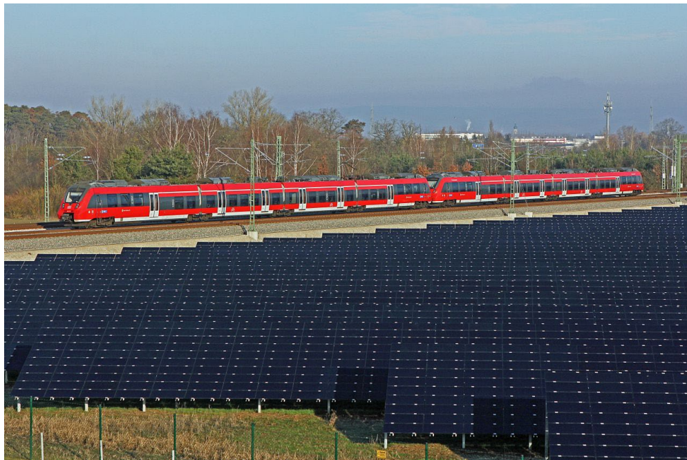
Photovoltaic system along a railway line © Deutsche Bahn AG / Photo: Claus Weber
