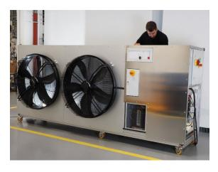
Demonstrator of a centrally installed external heat pump as a heating solution for apartment buildings. To date, there are only a few products with the natural refrigerant propane on the market for apartment buildings.
