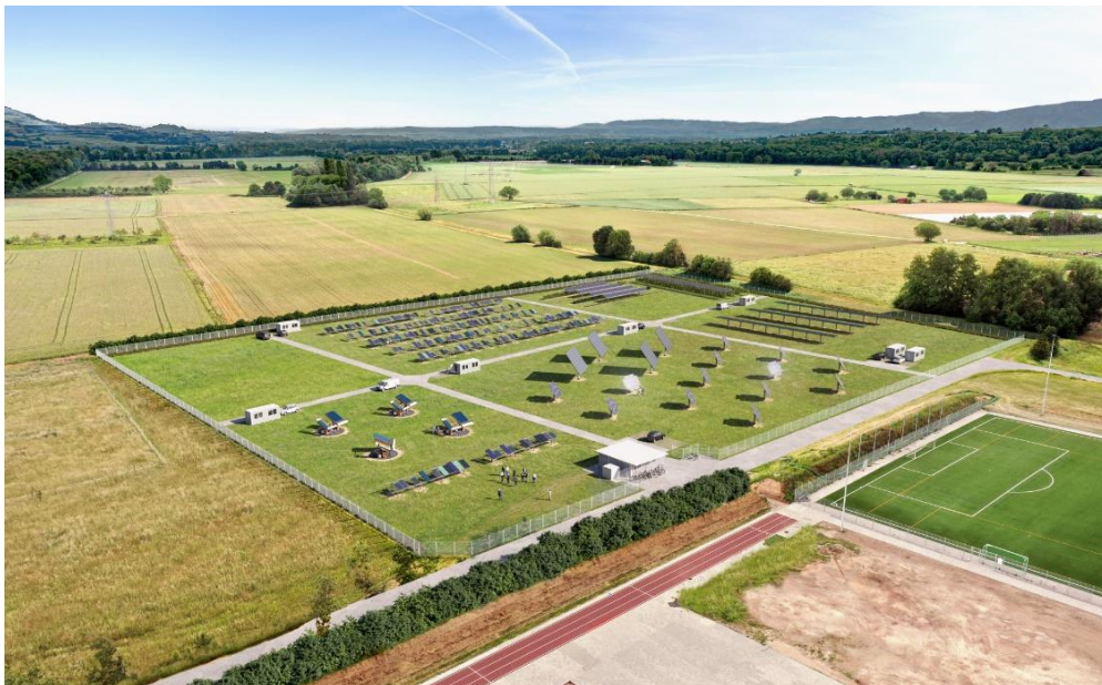
Visualization of the new Outdoor Performance Test Field in Merdingen, Germany as it may look in five years. © Fraunhofer ISE / Visualization: 3DLink
