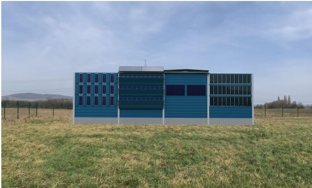
Rendering of four PV-integrated noise barrier elements, which are currently being installed at the Outdoor Performance Test Field of Fraunhofer ISE.
