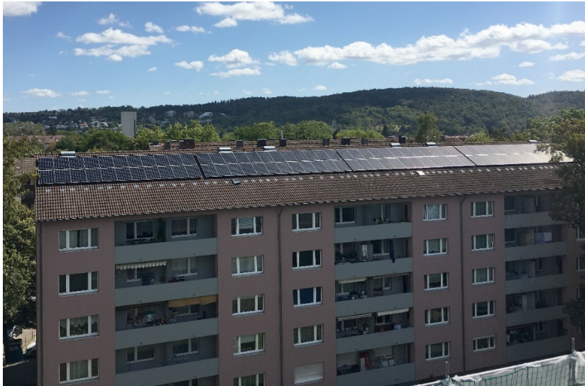
An apartment building in the Smart Quarter Karlsruhe-Durlach. A 60 kWp PV system was installed on the roof. © Fraunhofer ISE
