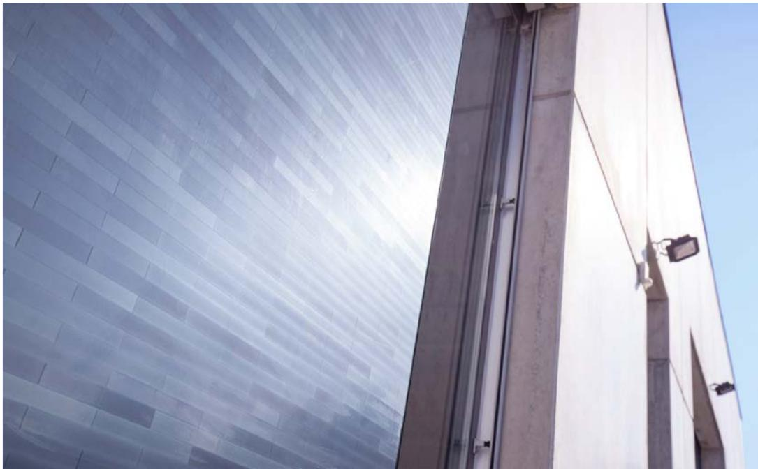
Matrix shingle modules are particularly suitable for integration into building facades with their high surface utilization, excellent performance under partial shading and aesthetic appearance. © M10 Industries AG
