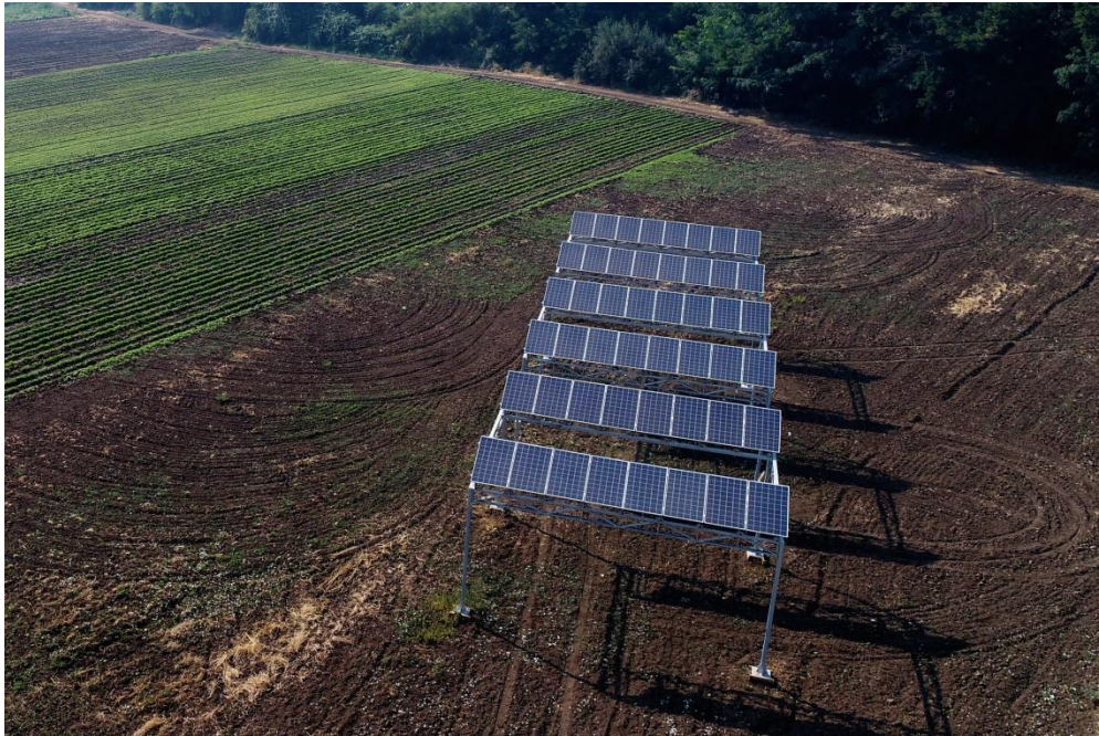
Each plant (here the one in Lampa) has a power of 13 kilowatts. ©Fraunhofer Chile
