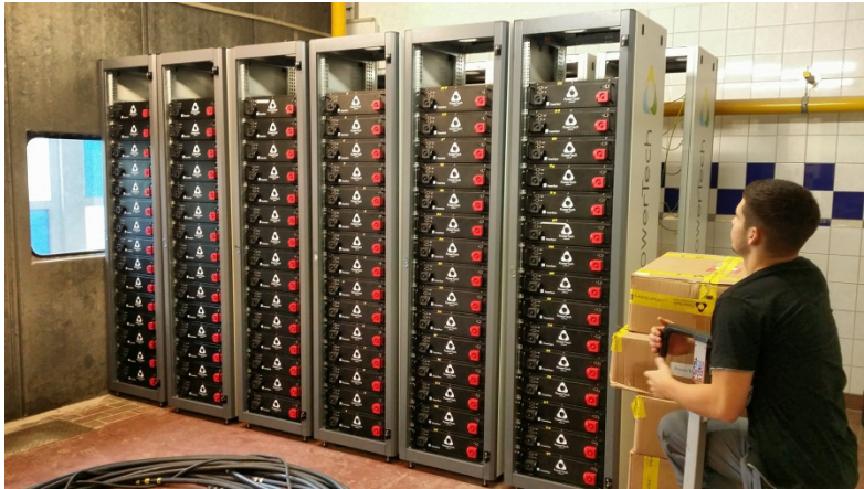
Installation of the battery storage system on the island of Borkum in Germany ©Fraunhofer ISE
