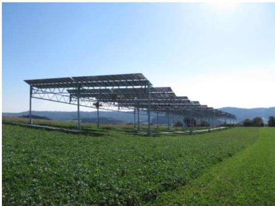
The PV plant with installed power of 194 kilowatts covers an area of one-third hectare. ©Fraunhofer ISE
