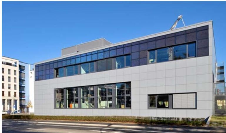
The Fraunhofer Institute for Solar Energy Systems ISE has integrated 70 PV modules of its own development and production into the building façade of one of its laboratories. ©Fraunhofer ISE
