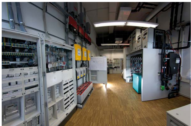
The SmartEnergyLab of Fraunhofer ISE: The digital agents are located in the three yellow cabinets. ©Fraunhofer ISE
