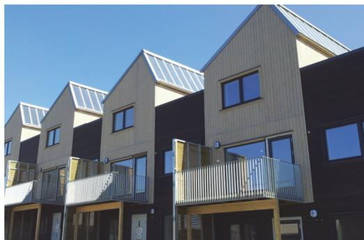
Terraced housing estate "Stenbråtli" near Oslo. Thirty-four terraced houses, built to passive house standards, were equipped with roof-integrated polymer solar collectors from the company Aventa. This system meets 60 percent of the total energy consumption of both the hot water and the space heating. ©Aventa
