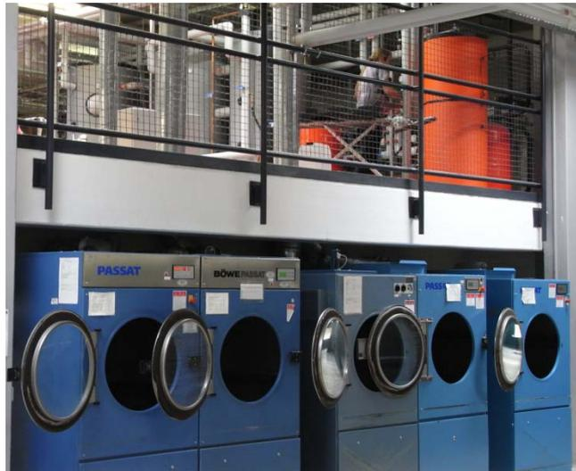
Fraunhofer ISE is developing a sector-specific concept for using solar heat in laundries, which involves solar thermal installations being integrated into the system to cover part of the heat required for individual processes. The photo above shows the storages of a solar thermal installation providing heat for boiler feed water, boiler make-up water and washing machines. ©Fraunhofer ISE
