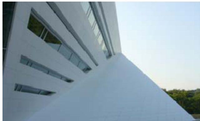
Detail of façade, Energy Dream Center in Seoul ©Fraunhofer ISE
