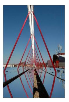
Fresnel collectors from Mirroxx on the roof of the University of Seville, Spain. The collectors provide process heat at a temperature of 180°C to drive a 2-effect absorption chiller for air-conditioning the building. ©Mirroxx GmbH
