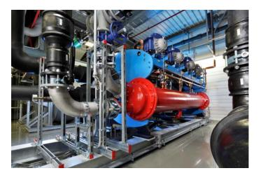
Heating and cooling with environmentally friendly energy dominates the energy efficiency concept at the Pfizer Manufacturing Deutschland GmbH facility in Freiburg. The chiller installed at the facility is shown in the photo. ©Pfizer Manufacturing Deutschland GmbH, Werk Freiburg
