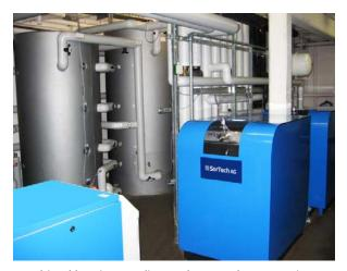
Combined heating, cooling and power demonstration system located at Fraunhofer ISE. Two adsorption chillers, each with a cooling power of 5.5 kW, use the waste heat from a CHP driven by natural gas. The end users are the scientists at Fraunhofer ISE, whose office rooms are heated and cooled by the system. © Fraunhofer ISE
