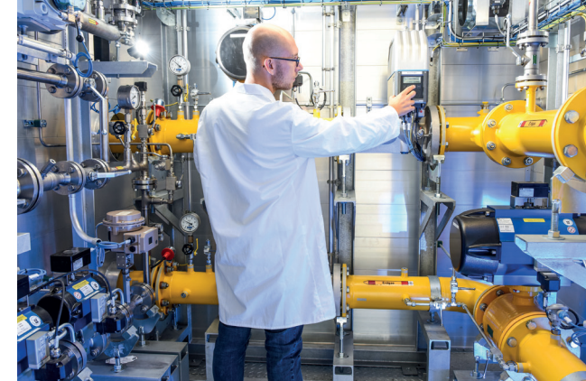
Institute's own hydrogen injection station into the local natural gas grid. We analyze, develop and optimize hydrogen infrastructures and supply chains.
