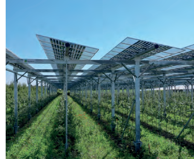
Research facility for agrivoltaic orcharding in midwestern Germany. © Fraunhofer ISE
