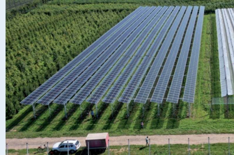
Apple orchard with agrivoltaic system in Gelsdorf, Germany with 258 kW p installed capacity.
