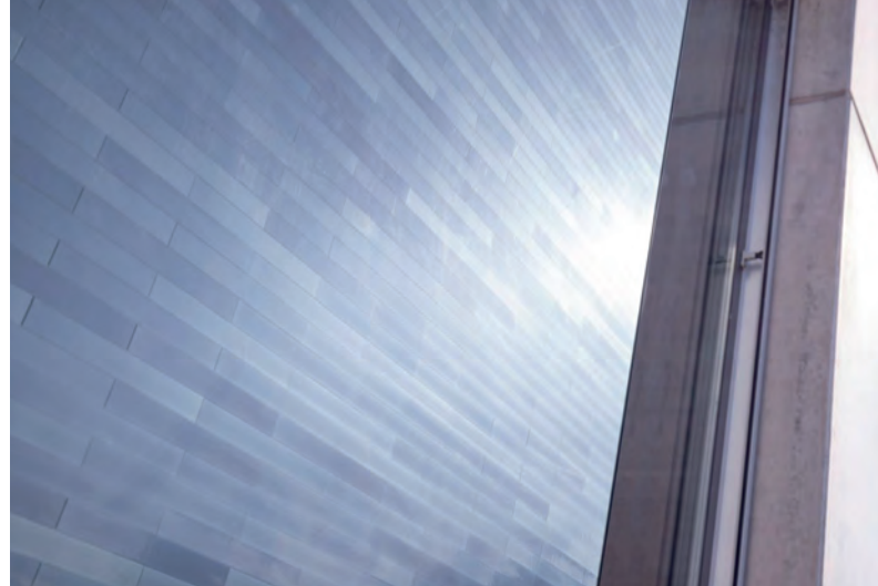
Matrix shingle modules installed as façade elements. © M10 Industries
