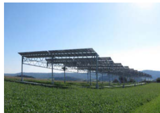
Figure 3: (System 2) 194.4 kWp APV system in Heggelbach, Germany.
