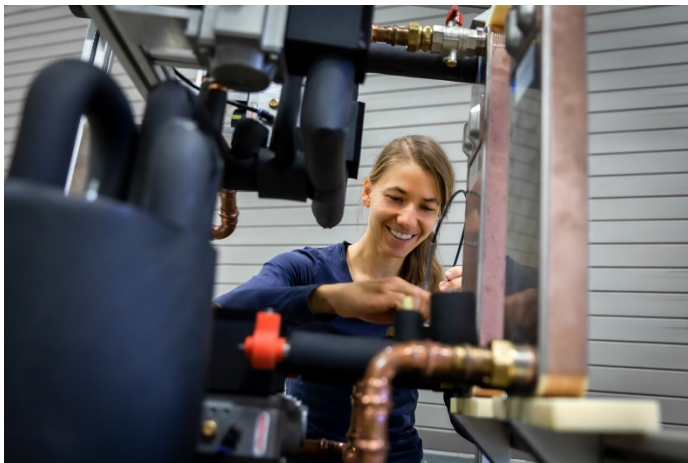
In the "LCR290" project, results from the "LC150" project are used to transfer refrigerant reduction to larger capacities in multi-family houses. ©: Fraunhofer ISE
