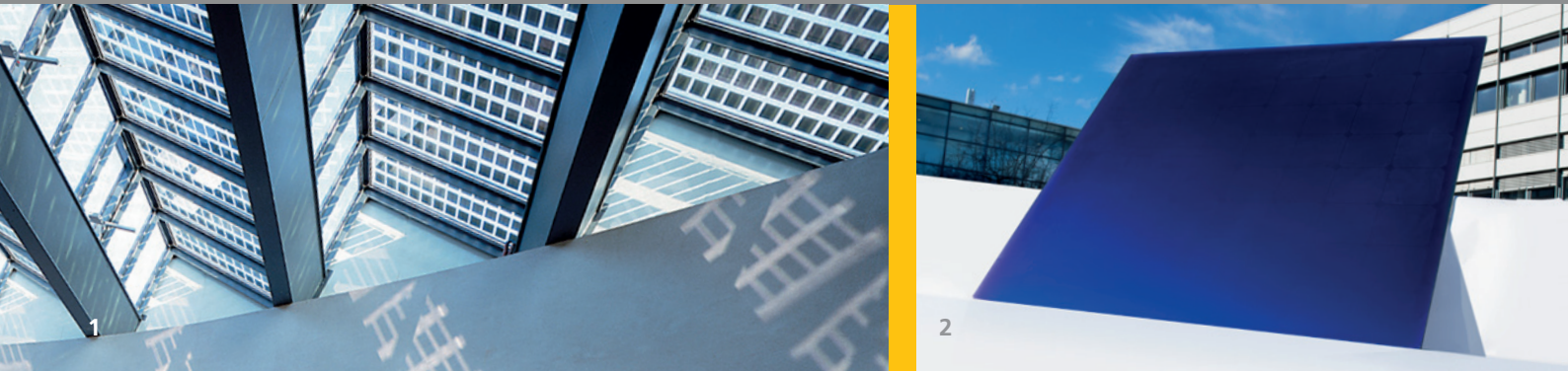
1 Semi-transparent BIPV modules integrated in a building of Fraunhofer ISE.
