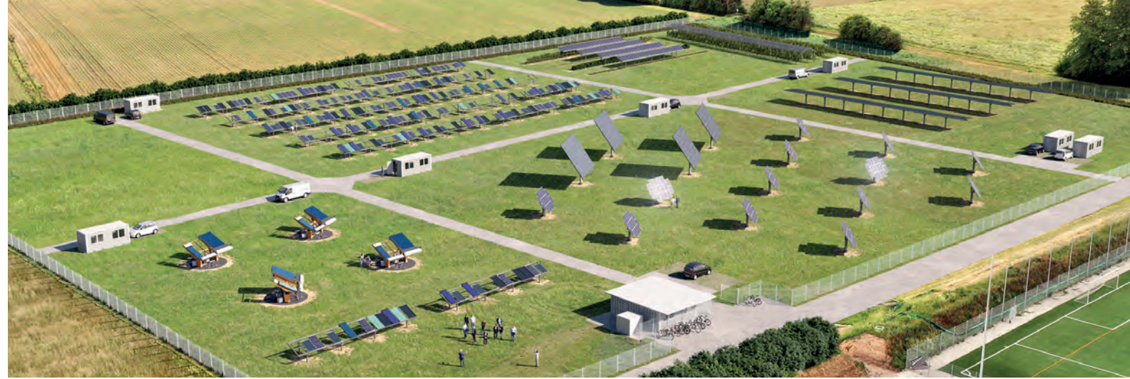
Visualization of the Solar TestField with different solar system setups in Merdingen near Freiburg, Germany.
