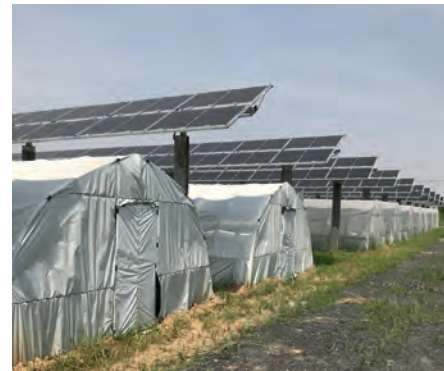
Fig. 45: PV modules above a polytunnel © BayWa r.e.
