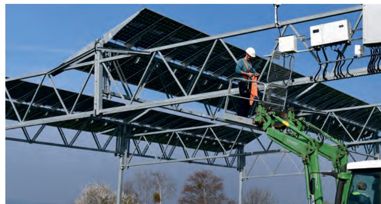
Fig. 60: Maintenance work on the agrivoltaic system in Heggelbach © Fraunhofer ISE
