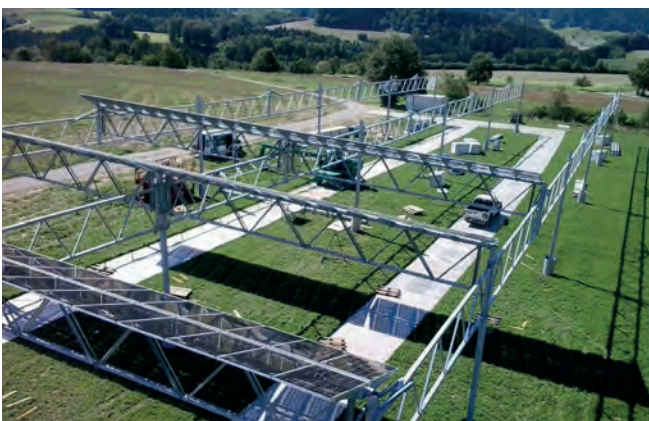
Fig. 59: Construction roads to avoid soil compaction © BayWa r.e
