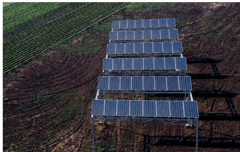
Fig. 23: Pilot PV systems in Curacaví and Lampa where the Fraunhofer Chile Research Institute is investigating which crops benefit from slightly less solar radiation © Fraunhofer Chile
