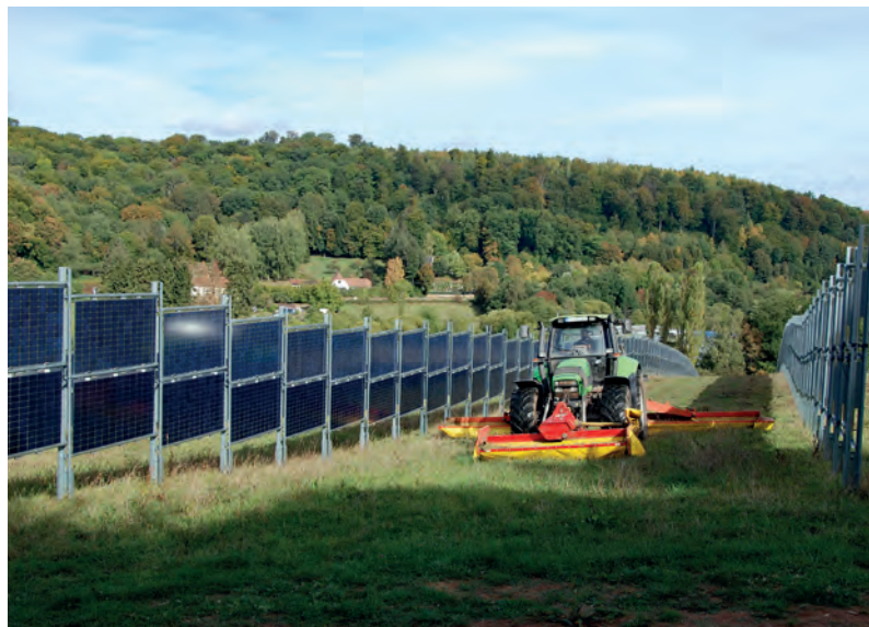
Fig. 36: Vertically deployed, bifacial PV modules used within the agrivoltaic system in Eppelborn-Dirmingen, Saarland, with 2 MW p of capacity, built by Next2Sun © Next2Sun GmbH
