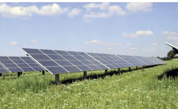
Fig. 7: Typical ground-mounted PV system © Fraunhofer ISE
