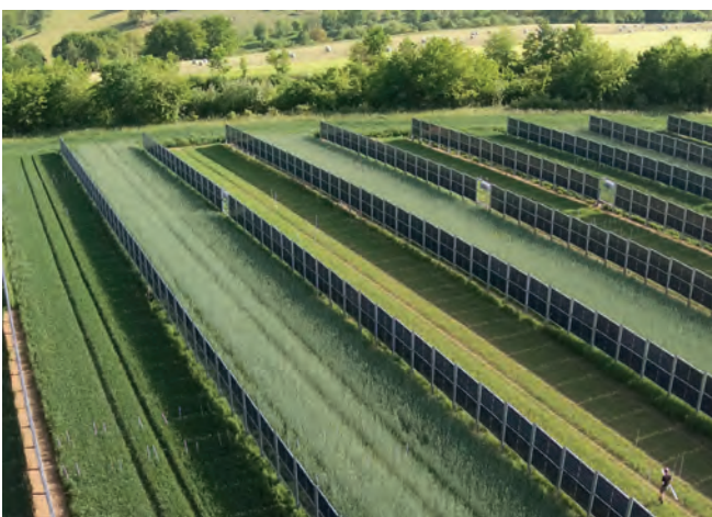
Fig. 22: Vertical agrivoltaic system in Merzig-Wellingen, 2023 © University of Hohenheim
