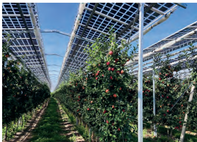
Fig. 21: Agrivoltaic system in Kressbronn (2022) © Fraunhofer ISE
