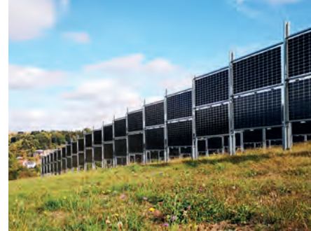
Fig. 44: Bifacial, vertically installed PV modules by Next2Sun, Eppelborn-Dirmingen © Next2Sun GmbH
