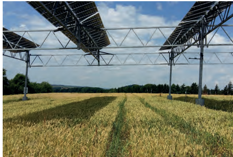
Fig. 53: The shaded strips underneath the PV modules move with the sun's position © University of Hohenheim
