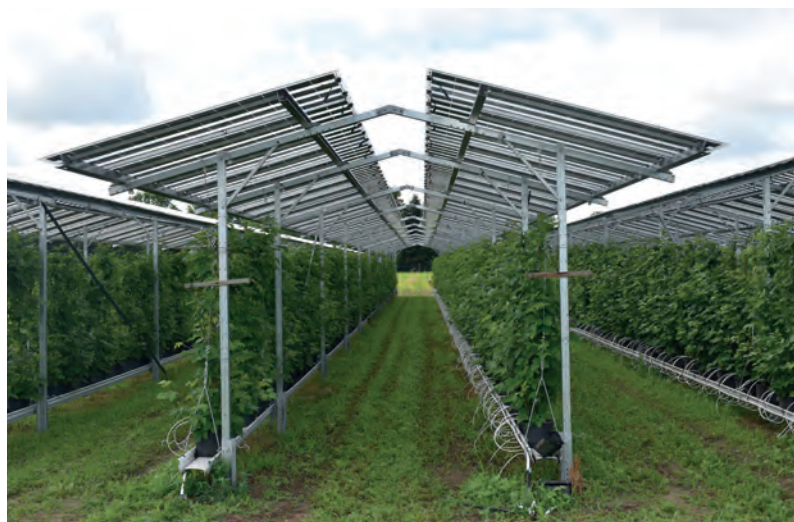
Fig. 43: PV modules with spatially segmented solar cells and protective function in the Netherlands © BayWa r.e.
