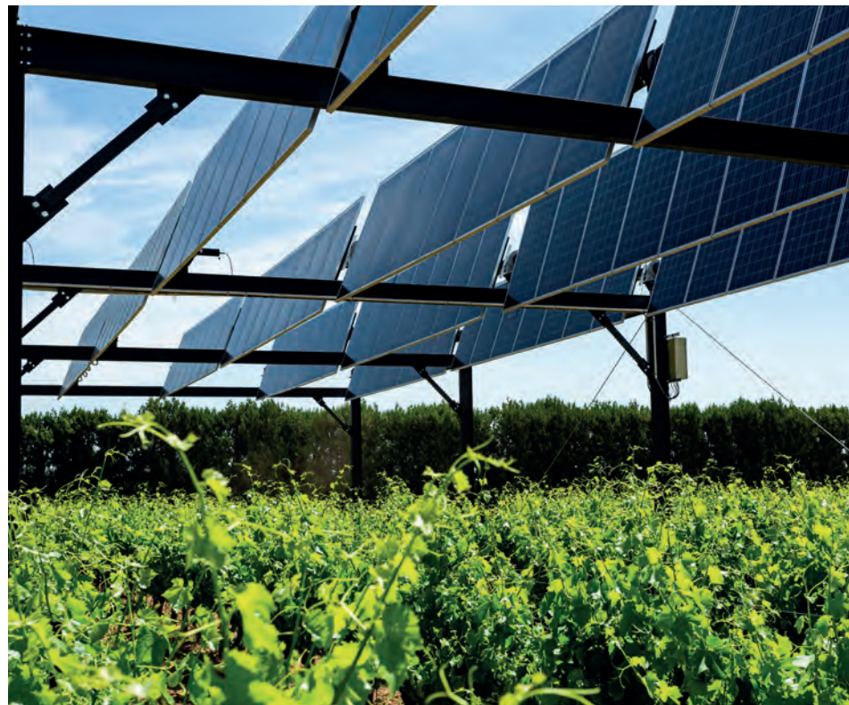
Fig. 50: Single-axis tracker system on a demonstration system in France © Sun'Agri
