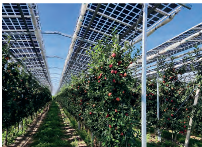
Abb.21: Agri-PV-Anlage in Kressbronn (2022) © Fraunhofer ISE
